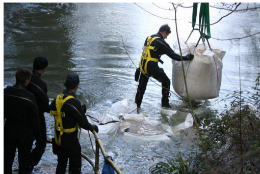
Army engineers lower gravel into the river Itchen, February 15 th
