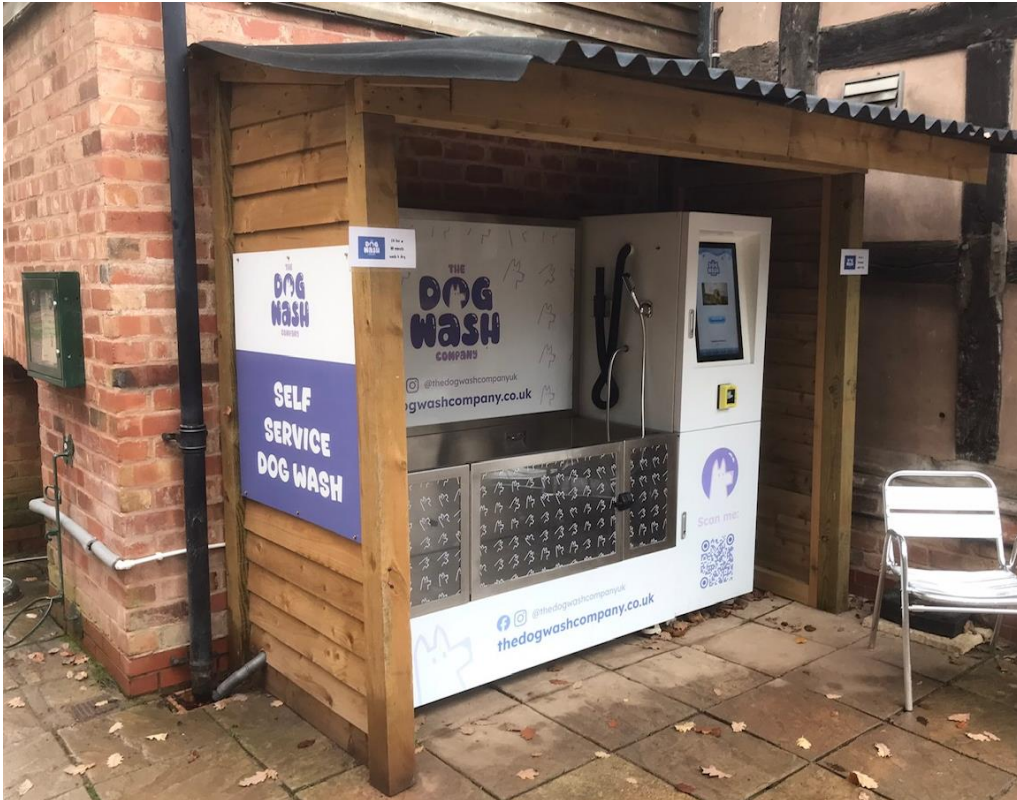
Figure 4. A Dog wash facility installed in a country park, with waste water emitting to the sewer at the bottom left of the photo.
